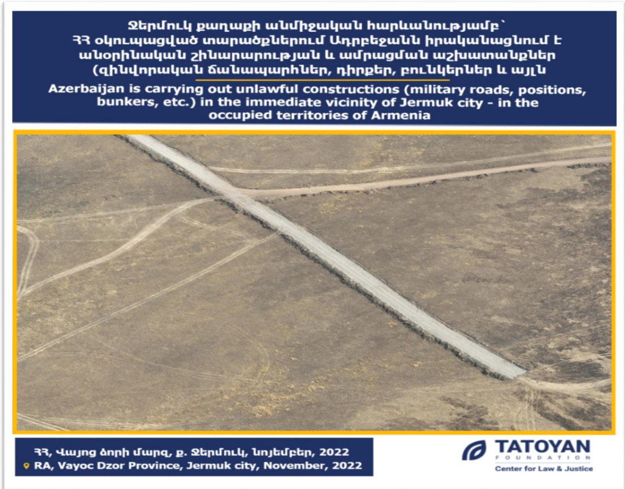
Figure 31: The road built in the occupied territories of the Republic of Armenia by the Azerbaijani armed forces; this area is in the immediate vicinity of Jermuk city, Vayots Dzor province.
